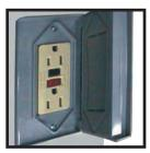
120V GFI duplex receptacle, located on the side of the panel, provides auxiliary power for other devices.
